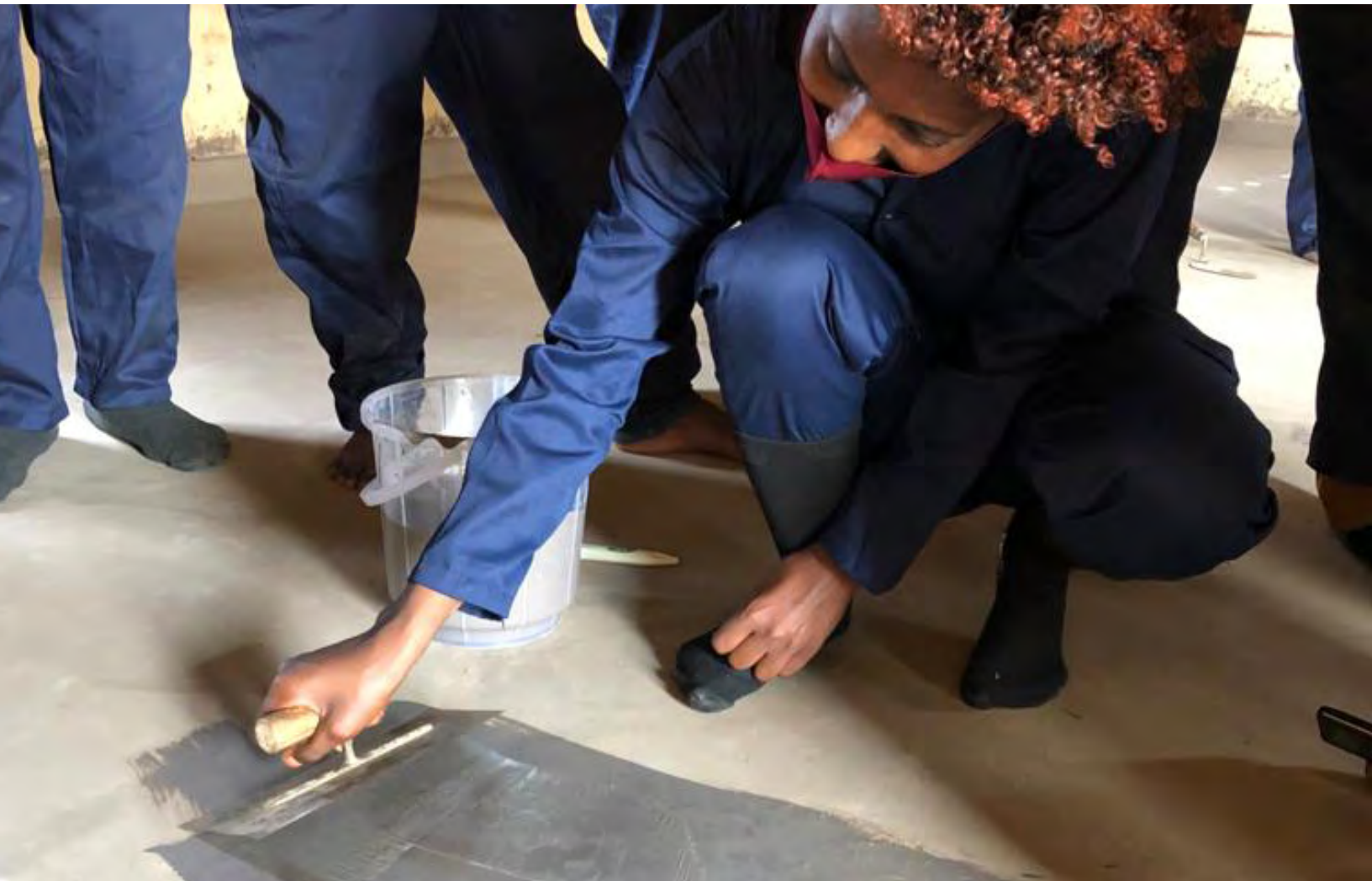
A mason demonstrates building an earthen floor. © EarthEnable
