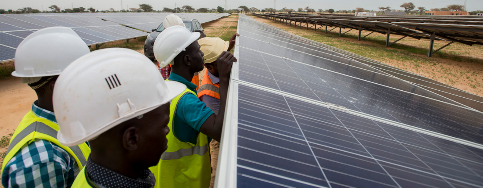
Inspecting solar PV panels at the Power Africa-supported Senergy I solar plant, a 29 MW facility that is currently the largest solar farm in West Africa. Photo: Xaume Olleros
