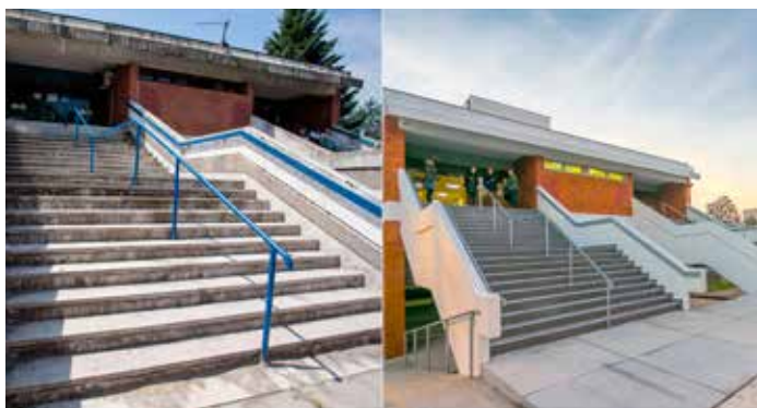
The USAID-funded renovation of the Belgrade Misdemeanor Court streamlined court operations, improved case management, and made it easier for citizens to pursue justice.
