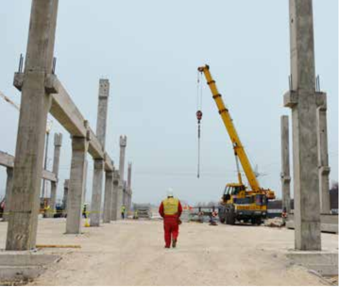
USAID supported the development and implementation of reforms in Serbia's construction permitting regime.
