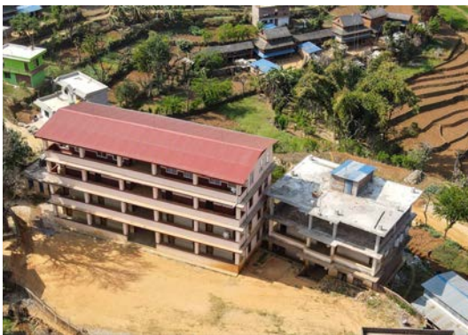
Lightning arrester installed on the rooftop of a school in Neelakantha Municipality. Credit: Tayar Nepal (2022)
