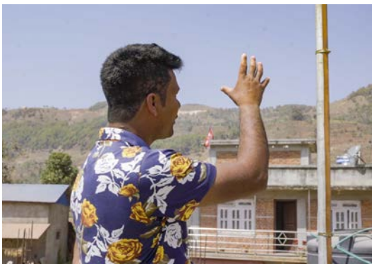
Electrician, Prakash Dhungana, showing the lightning protection system installed in Khatle's ward office. Credit: Tayar Nepal (2022)
