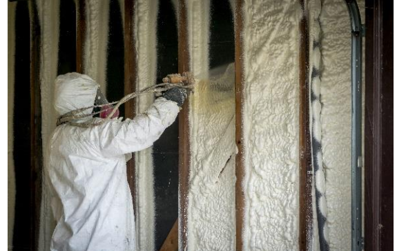
Figure 18. Rigid Polyurethane Spray Insulation
