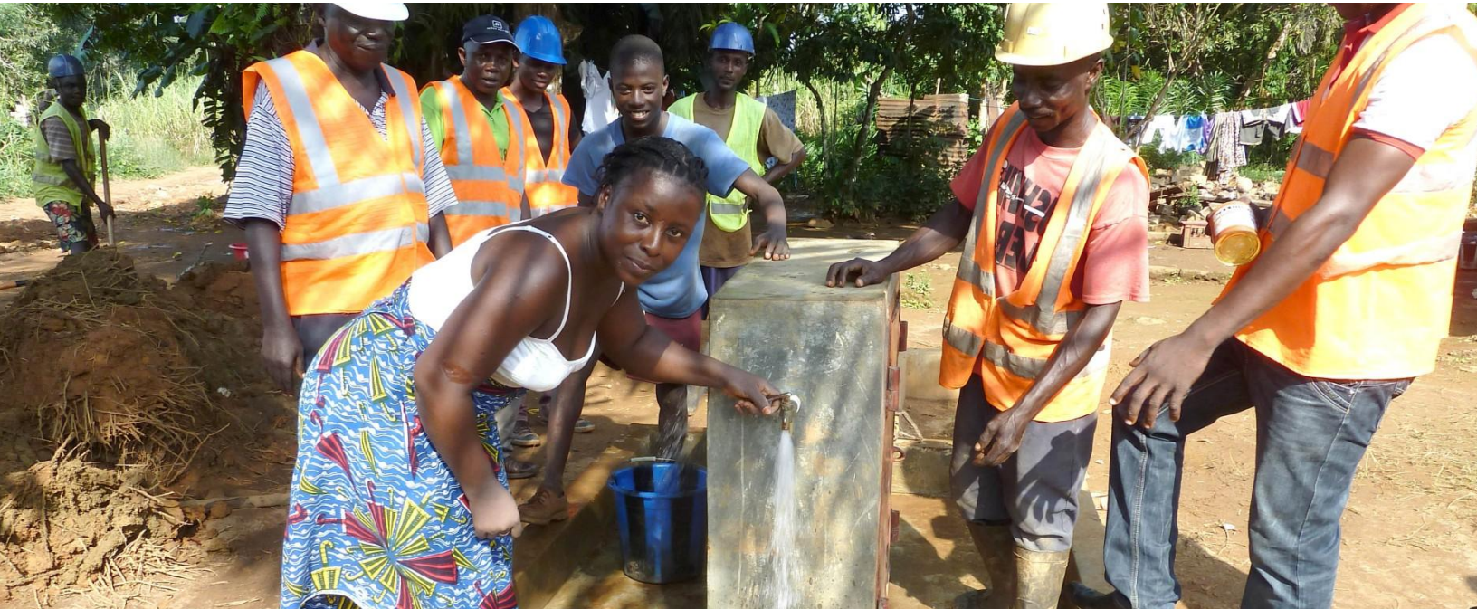
USAID LIBERIA MUNICIPAL WATER PROJECT / TETRA TECH
