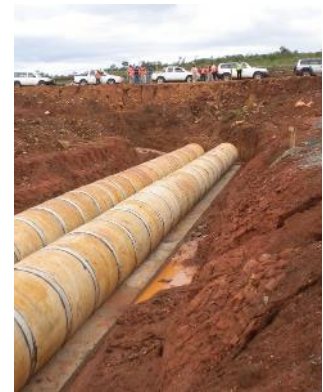
Figure 14. Double Pipe Culvert
