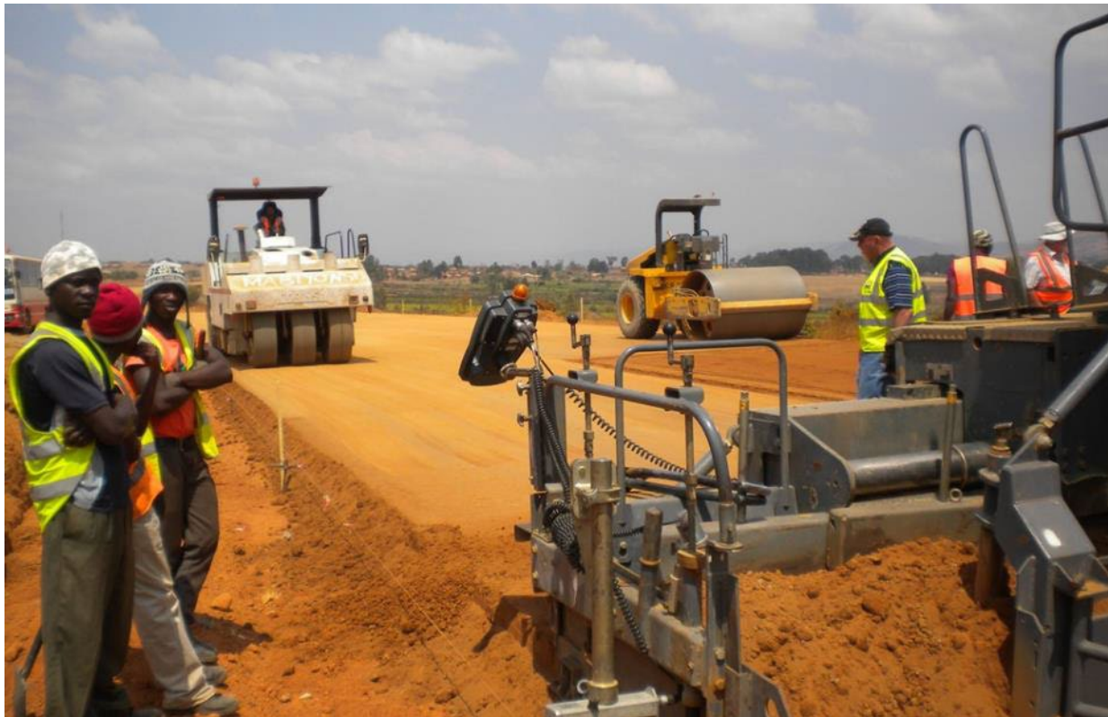
Figure 19. Compaction of Subbase Layer
