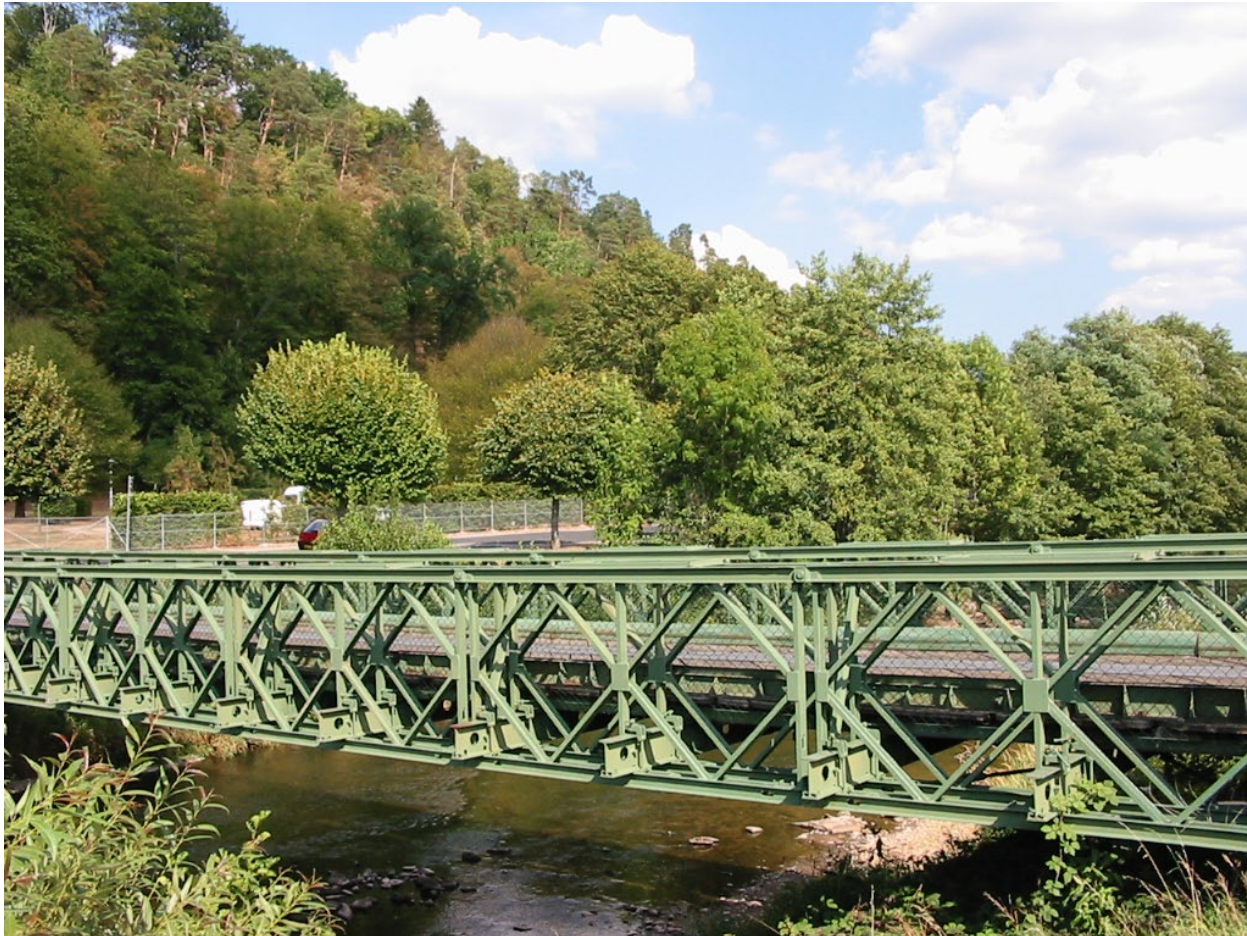
Figure 18. Bailey Bridge, Saint-Dié-des-Vosges, France
