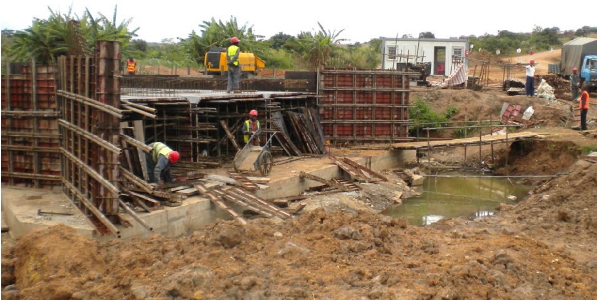
Figure 13. Concrete Box Culvert Under Construction
