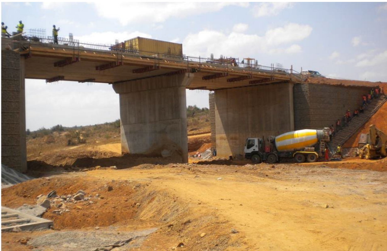
Figure 17. Concrete Bridge Under Construction
