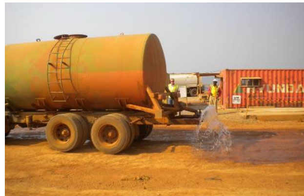
Figure 35. Water Truck Applying Water for Dust Control
