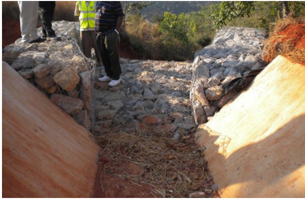
Figure 15. Gabion Outfall for Drainage Channel Discharge
