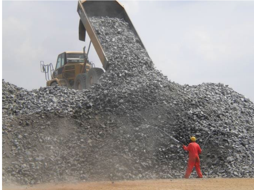
Figure 10. Stockpiling Crushed Rock
