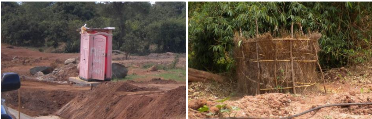
Figure 39. Temporary Pit Latrines
