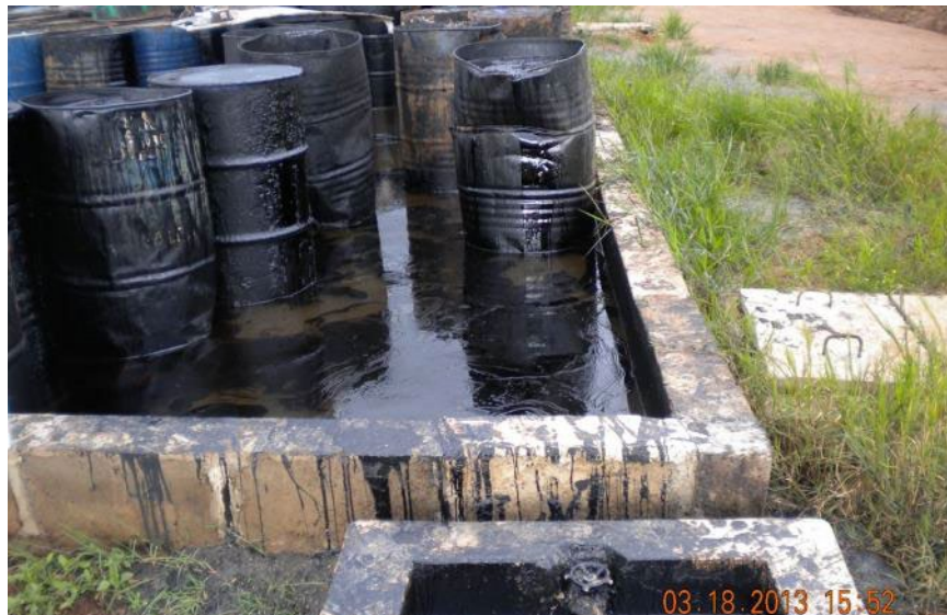
Figure 22. Leaking Bitumen Drum Storage with Secondary Containment
