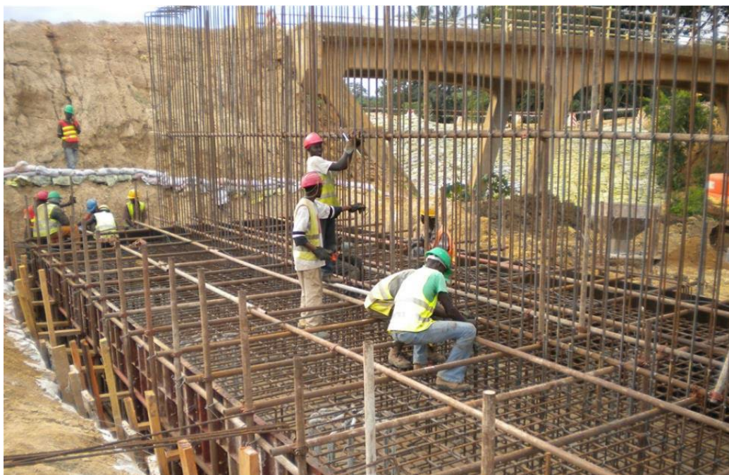
Figure 3. Placing Rebar for a Reinforced Concrete Bridge Pier
