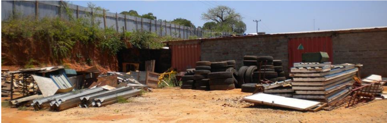
Figure 36. Temporary On-Site Storage Area for Construction Waste
