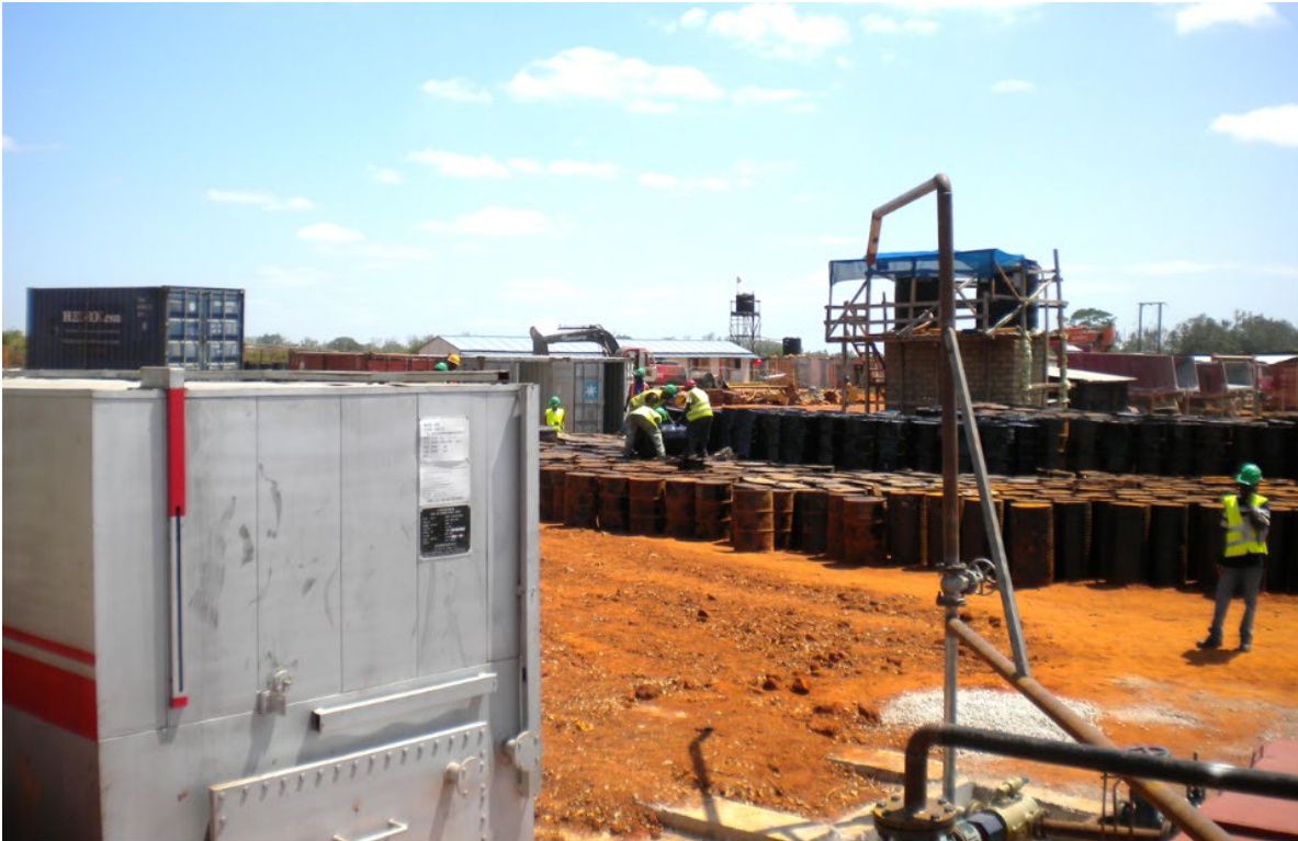
Figure 6. Material Laydown Area
