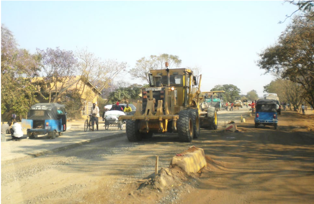
Figure 12. Half-Width Road Construction
