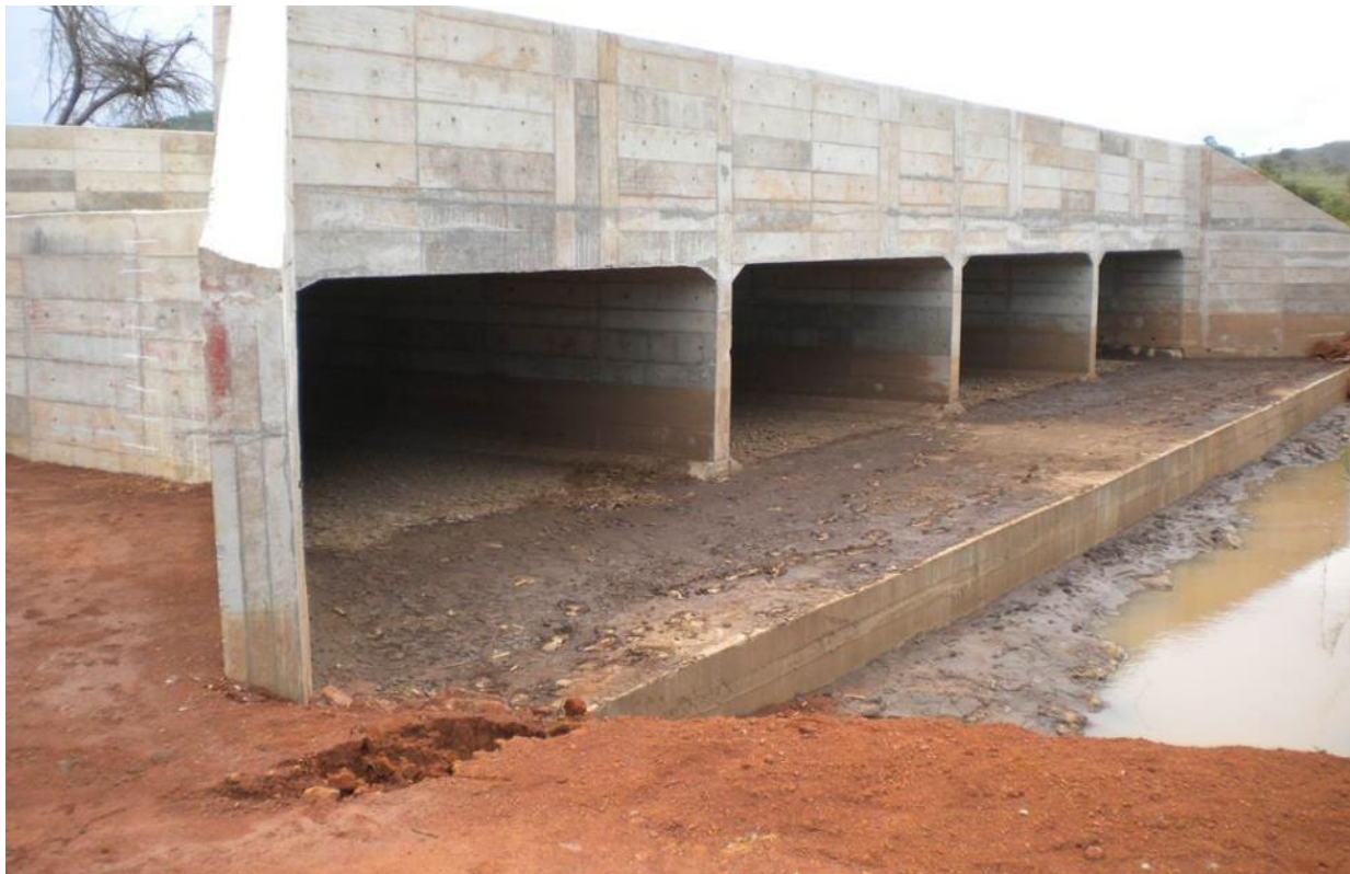
Figure 16. Multi-Section Box Culvert
