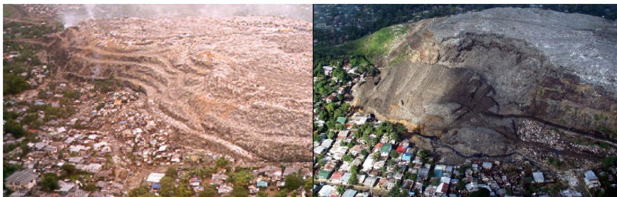
FIGURE 10. PAYATAS LANDFILL COLLAPSE – BEFORE AND AFTER 72
